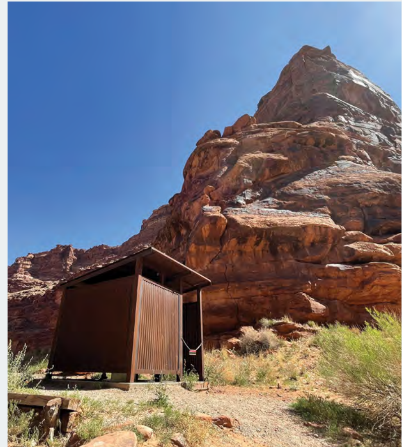
Figure 3-009—The pattern and colors in the weathered steel used here reflect the rocks and boulders of the setting and reinforce scenic character.
