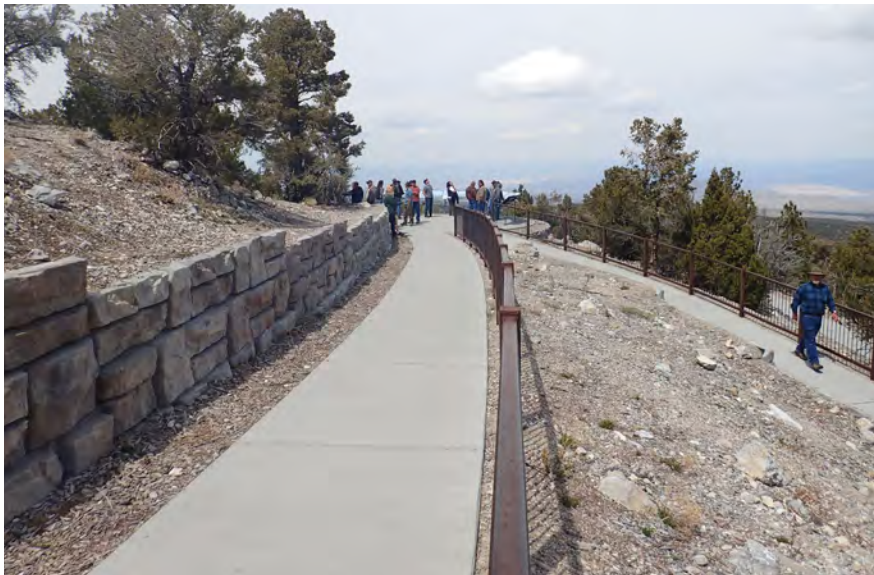
Figure 4-061—Creating an accessible route may require construction of retaining walls, but these should not fundamentally alter the character or function of the site.
