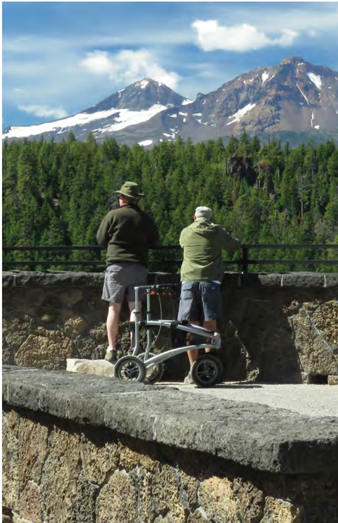
Figure 4-065—Local construction materials complement the natural scenic character. Rock walls have a high initial cost but a low lifecycle cost. Dark-colored railings protect visitors from the edge while reducing visual contrast with the surrounding landscape.
