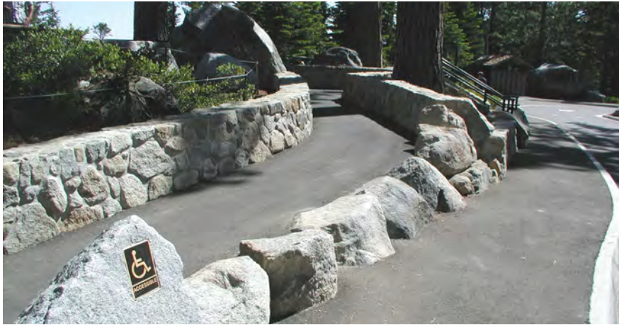
Figure 4-060—Design paths to respond to natural topography and site character. Careful design of the route to a viewing area constitutes part of a high-quality experience for visitors.
