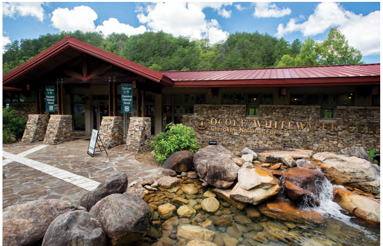
Figure 3-022—Pay careful attention in the design to the way a building meets the ground. Depending on the locality, naturally shaped and weathered stone placed near the base of a structure helps to visually anchor it to the landscape.
