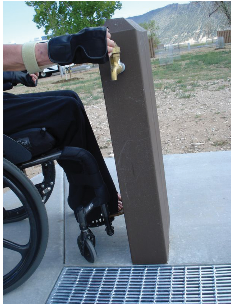
Figure 3–104—Select water spigots with universal design principles. The water spigot lever handle should be operable with a closed fist. The surface should be firm and stable, with enough space so that a person using a wheelchair can maneuver behind the faucet to avoid splash from the hydrant.
