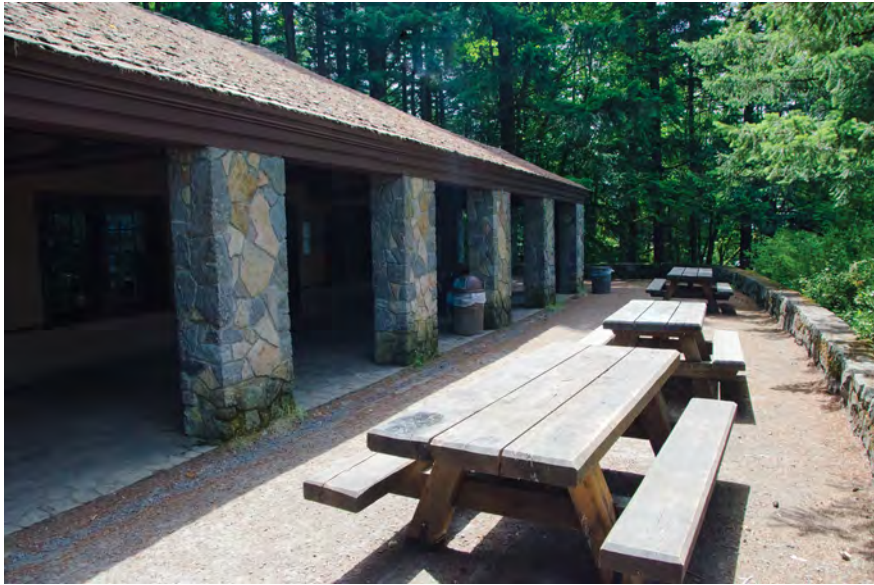
Figure 4-048—Picnic tables outside a visitor or interpretive center offer a valued amenity and can expand the time that people stay at the site.
