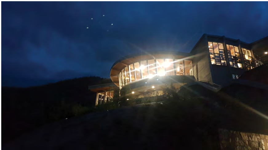
Figure 3-096—Shield lights in and around buildings from shining up into the sky. This photo is of the Mendenhall Glacier Visitor Center, Tongass National Forest.
