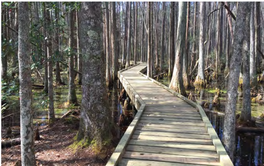
Figure 3–085—Elevated boardwalks can protect sensitive soil and riparian areas while providing sustainable visitor access. These features are relatively expensive to construct and require routine maintenance.
