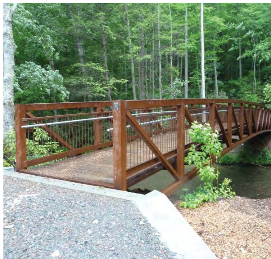
Figure 3–054—This stream crossing accommodates the 100-year flood level and provides aquatic organism passage.
