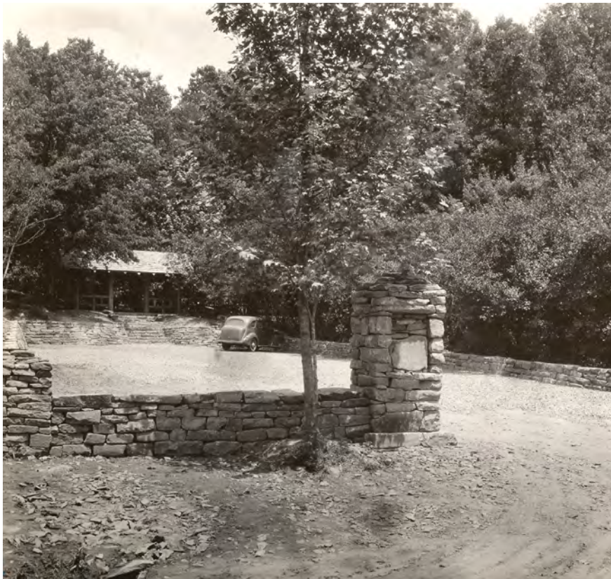
Figure 1–008—Extensive rock work was a common element of Civilian Conservation Corps recreation sites.
