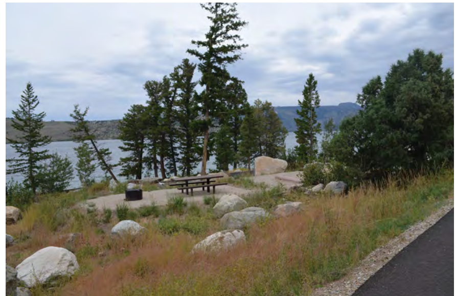
Figure 4–003—Many Forest Service campgrounds constructed decades ago (top) require renovation to bring them to current standards (bottom).
