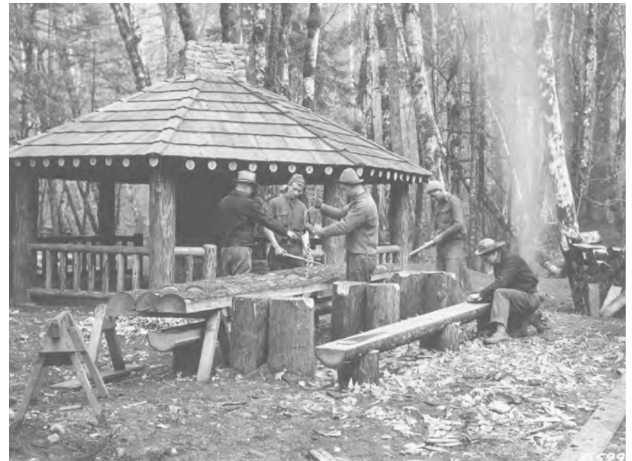
Figure 1-007—A Civilian Conservation Corps team constructing a picnic pavilion from materials found onsite.
