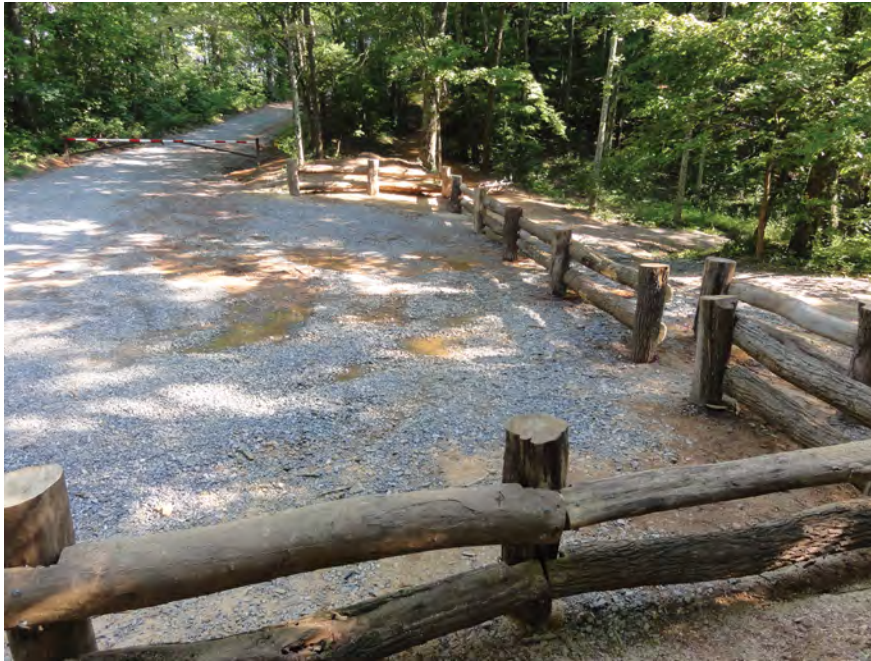
Figure 3–035—Naturally tapered wood and rough-sawn lumber elements help reinforce local scenic character.
