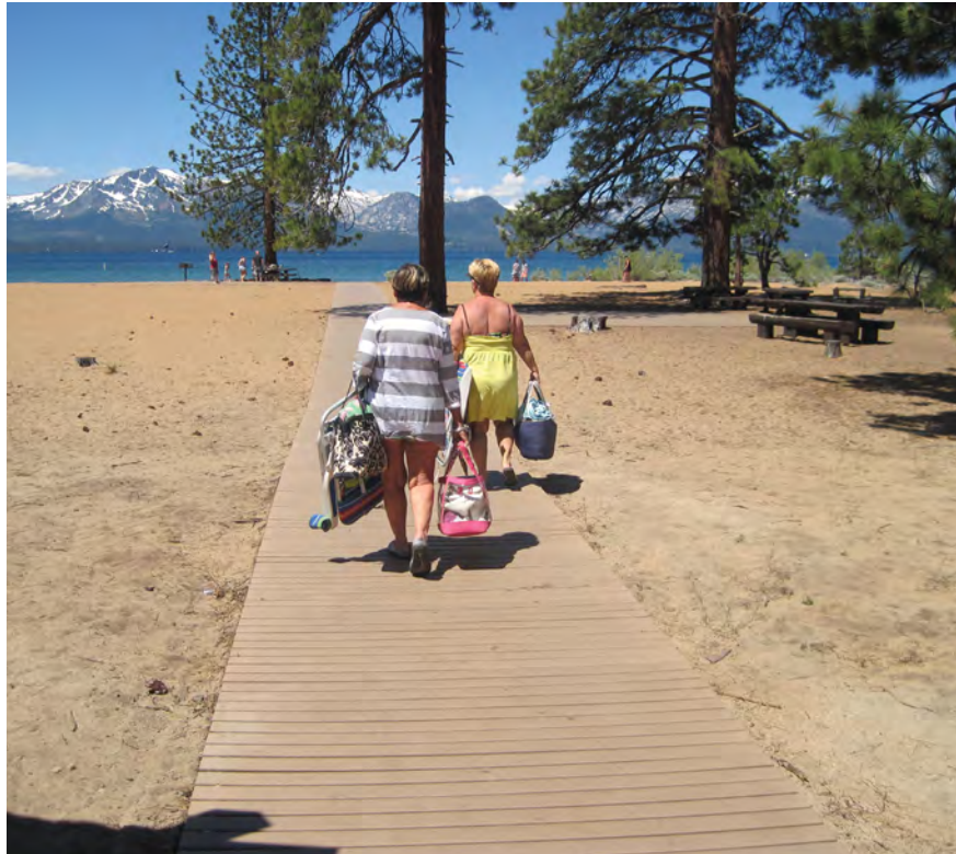
Figure 4-093—Providing accessible travel routes to swimming areas can present a design challenge. In this example, recycled plastic lumber is cabled together and lays directly on the sand to form a firm, stable surface.
