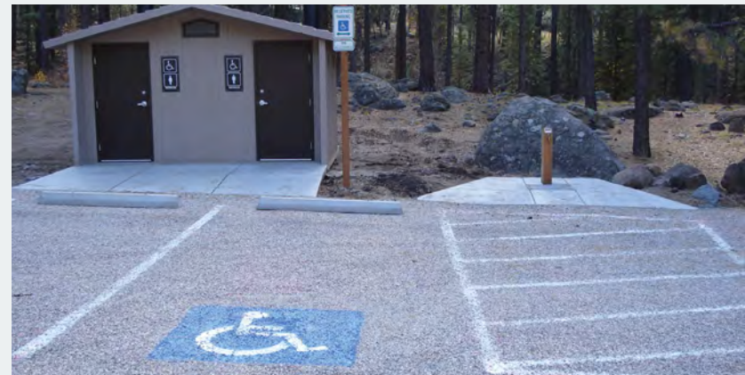
Figure 3-060—Identify accessible parking spaces using the international symbol of accessibility. Refer to the Architectural Barriers Act and the Forest Service Outdoor Recreation Accessibility Guide for requirements on painting asphalt.
