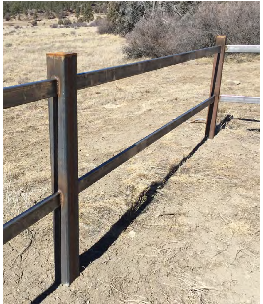
Figure 3–121—Self-weathering steel reduces contrast by oxidizing into colors found in the environment. While initial costs may be higher than other materials, self-weathering steel lasts a long time and has low maintenance requirements.
