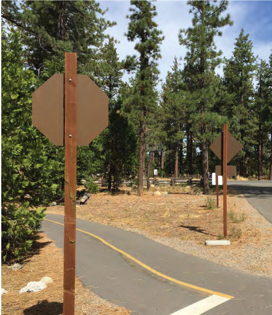
Figure 3–038—Painting the backs of metal signs reduces impacts of visual contrast and improves the visitor experience.
