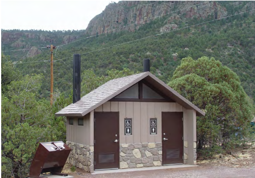
Figure 3–033—Use concrete color and texture to help development fit into its surroundings.
