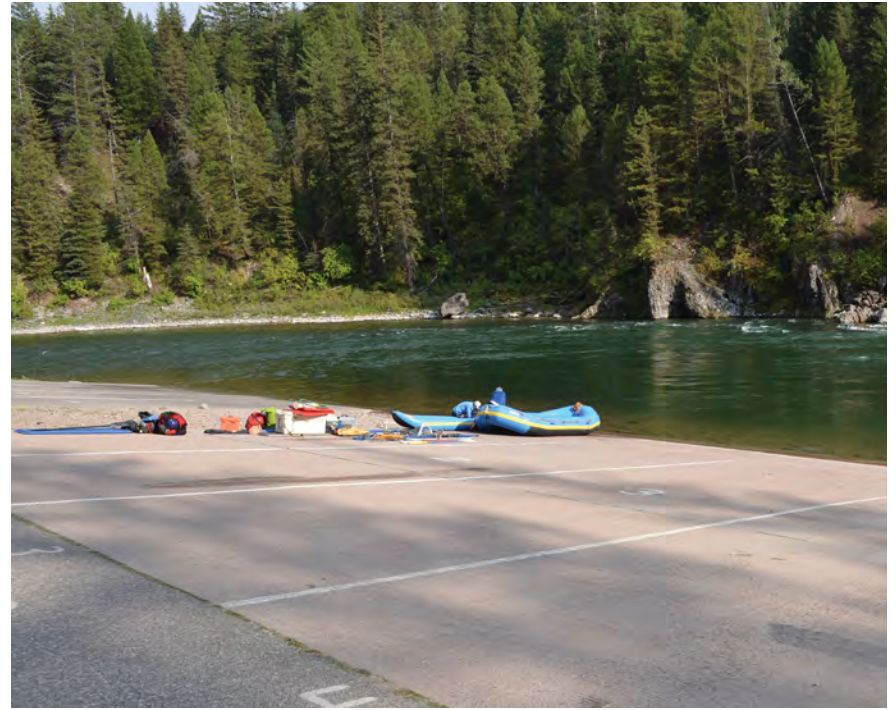
Figure 4-088—High-use boating facilities may require multiple launch lanes to accommodate the use levels.
