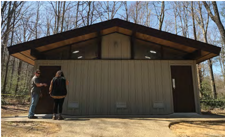
Figure 3–098—Incorporating skylights (top), including those that direct sunlight to ceiling-mounted lenses (bottom), can increase building functionality while reducing electricity consumption.
