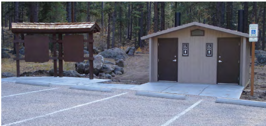
Figure 4–027—Clustering visitor amenities such as a kiosk and restroom can aid in providing accessible facilities.
