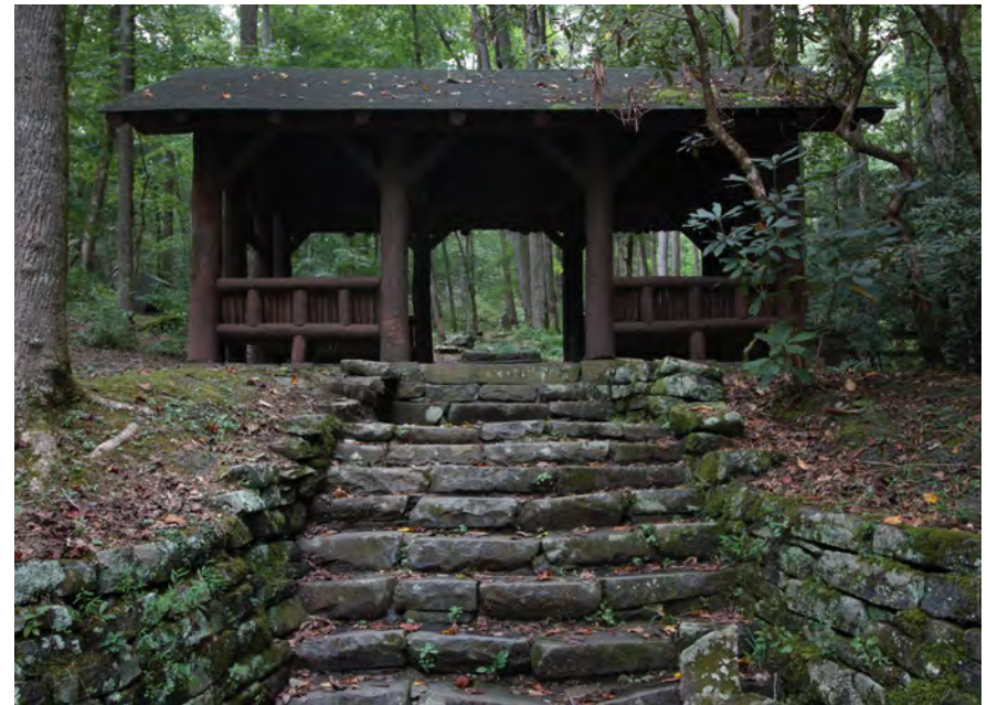
Figure 3-021—Retaining walls and steps respond to site topography and help reinforce site character.
