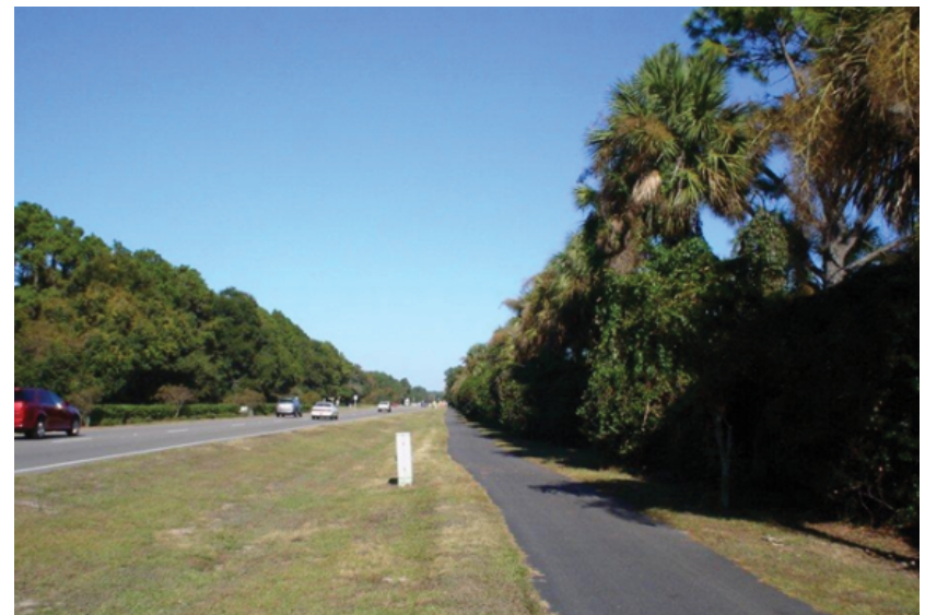
Figure 3–010—Burying electrical and communication wires underground improves scenic quality and reduces risks from wildfires. Photo credit: Scenic America.
