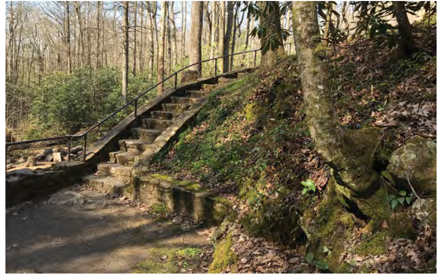
Figure 4-062—Steps, although not accessible, can allow retention of the natural character of the setting. In this case, the stairs are visible from the parking area. Where stairs have been included in the path but are not visible from the parking area, include a sign with a map to the overlook to help visitors make an informed decision about whether to attempt the path.
