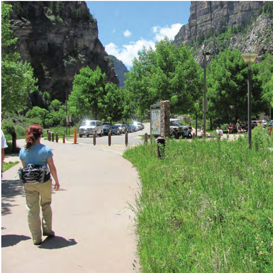
Figure 3–080—Stormwater runoff can be directed to areas for infiltration and support of vegetation.
