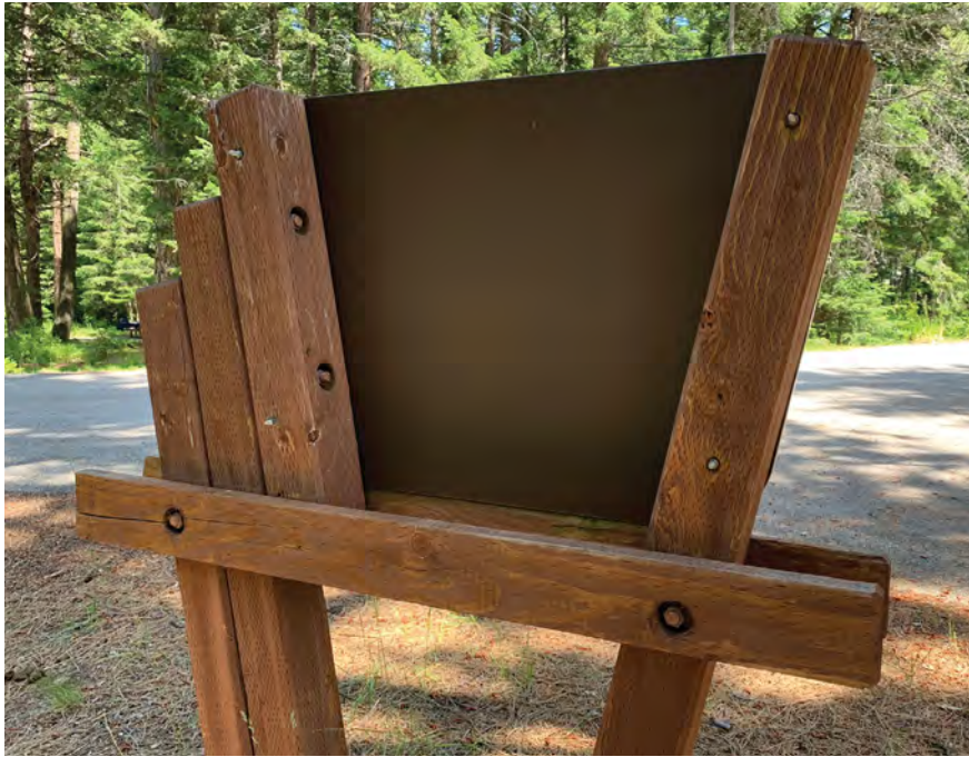
Figure 3-117—Paint or treat the backs of signs to reduce contrast and improve the visual quality of sites.
