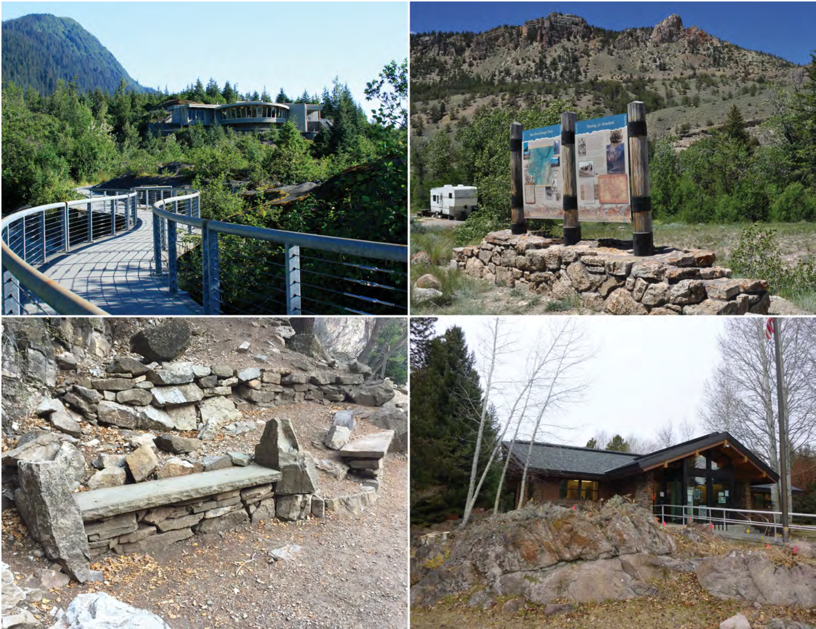
Figure 3-119—The form of constructed features should harmonize with the setting.
