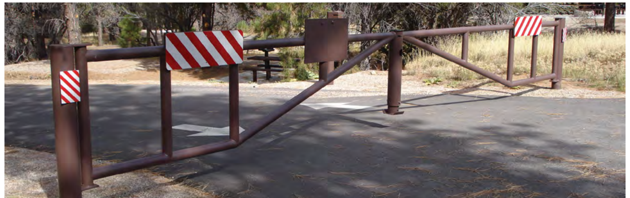
Figure 3-050—Provide gates to enable closure of the site or portions of the site to public access.
