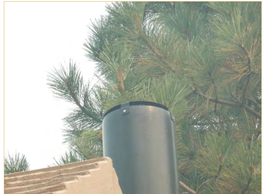
Figure 3–107—To reduce risks to birds and bats, install vent screens over vault toilet stacks.
