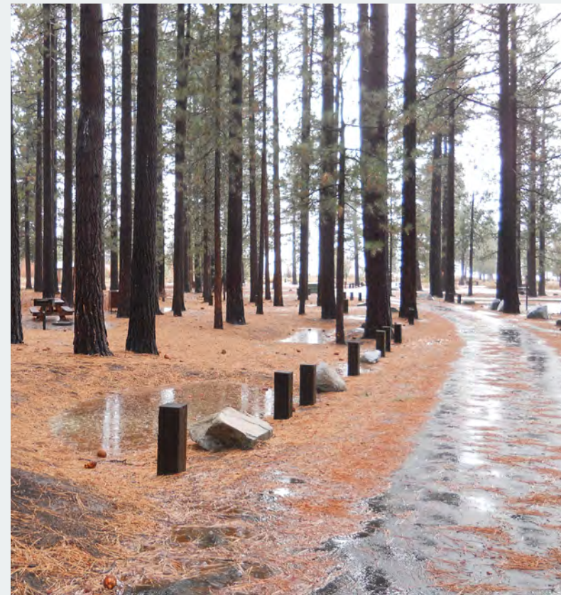
Figure 3–082—Direct and distribute stormwater to areas where it can infiltrate, as shown in this example of campground microbasins.
