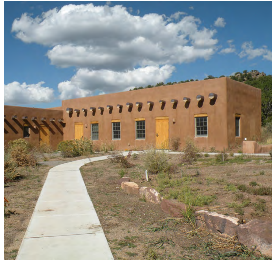
Figure 3–039—In the desert Southwest, adobe construction, a traditional building practice in the region for hundreds of years, keeps building interiors cool in the summer and warm in the winter. This material also complements the area’s scenic and cultural character.
