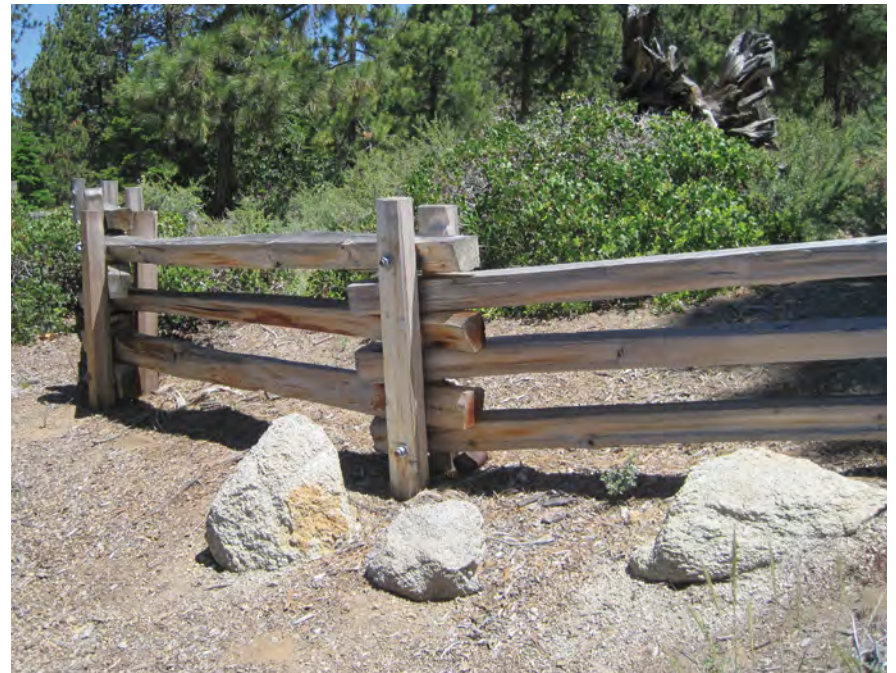
Figure 3–032—This durable, heavy-gauge, split-rail fence material promotes the site's rustic character.
