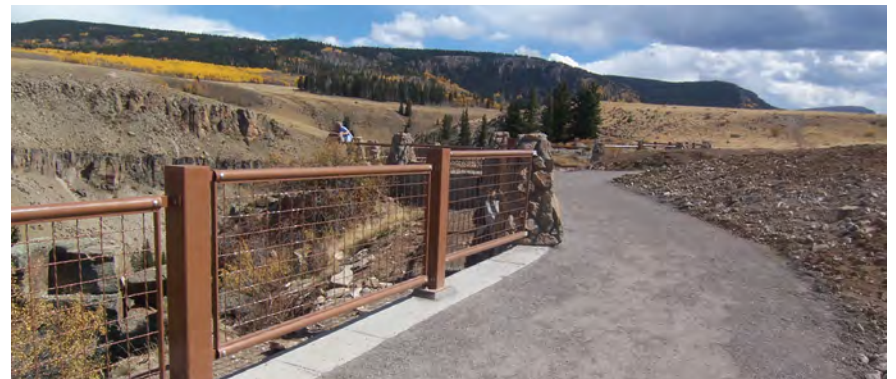
Figure 4-063—An elevation difference of 30 inches or more requires installation of 42-inch-high guardrails with openings of no more than 4 inches. The design of this guardrail minimally intrudes on the view, allowing views for visitors who may not be able to see over the top of the rail.
