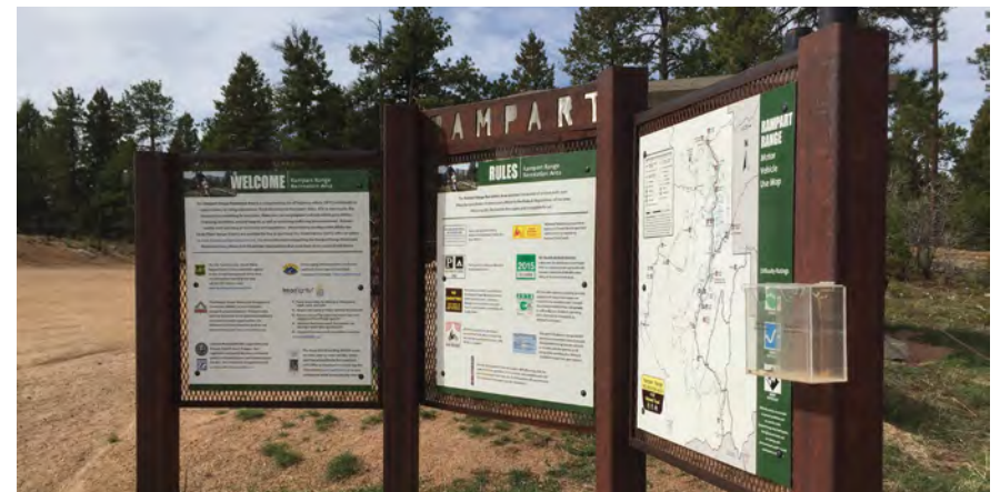
Figure 3–126—Durable, self-weathering steel sign frames often require far less maintenance than wood but cost more for materials, manufacturing, and installation.
