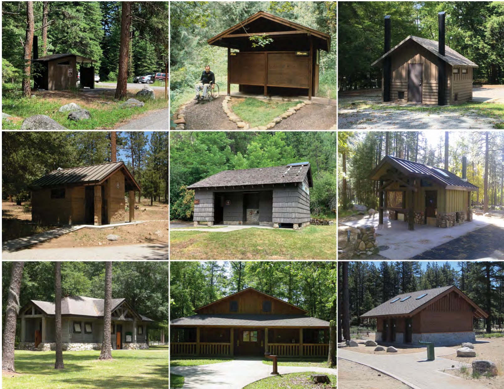
Figure 3-105—Toilet buildings, often the only building at Forest Service recreation sites, represent an important opportunity to express how the built environment should relate to its setting.
