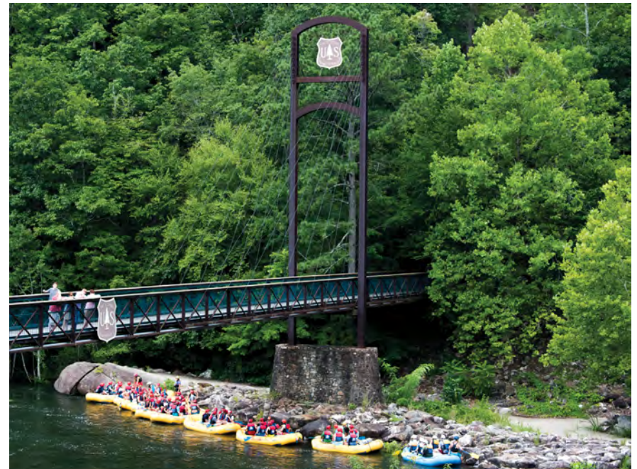
Figure 3–037—Long-lasting, self-weathering steel requires little maintenance and generally complements its surroundings.
