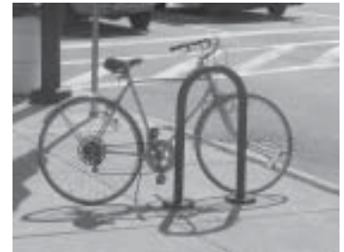
Select bicycle parking devices according to the need of the users and level of security required: 1) lockers for long-term secure storage, 2) racks that secure the frame and wheels for mid-term storage and 3) leaning rails for short-term low-security storage.
