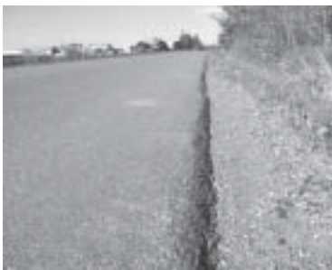
When roads are resurfaced, raise the level of the adjacent unpaved shoulder flush with the new roadway surface. Otherwise, a vertical drop onto a low shoulder can cause a bicyclist trying to ride back onto the roadway to fall into the path of overtaking vehicles.
