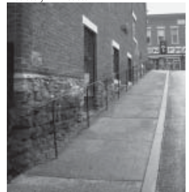
A handrail attached to a building can help pedestrians more comfortably negotiate sloping sidewalks.
