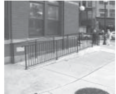
Parallel ramps can facilitate access to buildings where raised entrances were originally constructed with steps.
