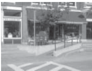
Mid block ramp with handrail.
