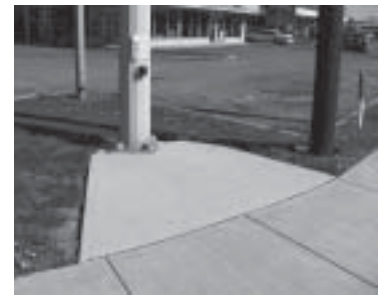
Use the same material in front of a pedestrian signal control as is used for the adjacent sidewalk or path.
