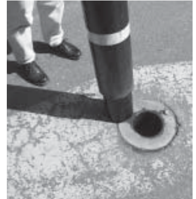
. . . but need to be designed to permit access for maintenance and emergency vehicles.
