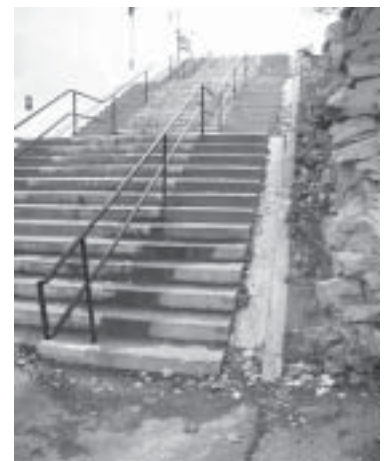
Where bicyclists need to change elevation using a stairway, provide a groove wide enough to accept a bicycle tire along the top of the stringer on both sides of the stairway.
