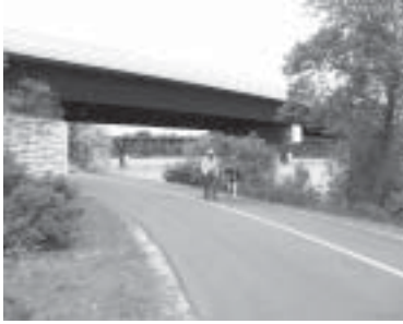
A vertical clearance of at least 3 m (10 ft) is preferred for undercrossings.
