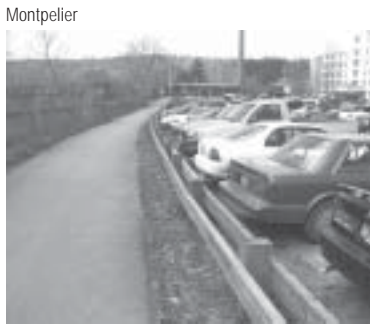
A shared use path may be delineated from a driveway, parking lot or other improved surface through the use of guardrail, fence or low landscaping.
