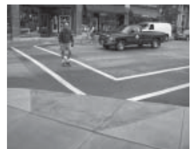
Diagonal curb ramp
