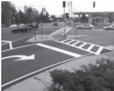
Well-designed slip lanes provide pedestrian crossing islands within the intersection and optimize motorists’ view of pedestrians.
