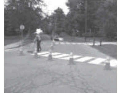
Regularly inspect and repaint crosswalk markings as required.
