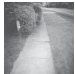
Clear vegetation that encroaches upon or restricts the use of a pedestrian walkway.
