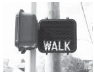
Existing pedestrian signal indications with lettered messages may be retained for the remainder of their useful service life.
