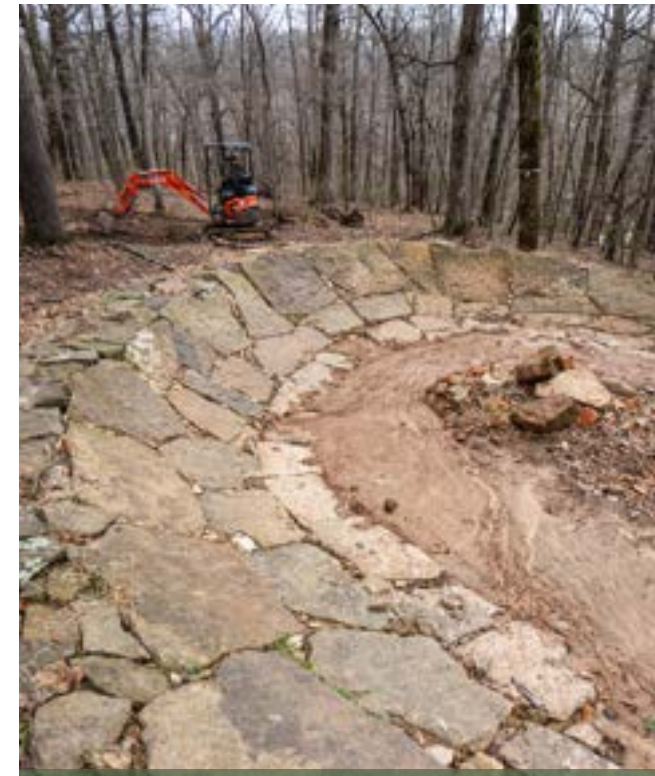
Rock berm under construction on the Boo Boo trail at Slaughter Pen in Bentonville, Arkansas. Photo by Kyle Copeland/Rock Solid
