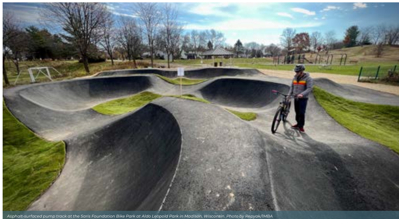
Asphalt-surfaced pump track at the Saris Foundation Bike Park at Aldo Leopold Park in Madison, Wisconsin. Photo by Repyak/IMBA
