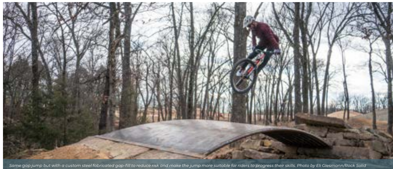
Same gap jump but with a custom steel fabricated gap-fill to reduce risk and make the jump more suitable for riders to progress their skills. Photo by Eli Glesmann/Rock Solid
