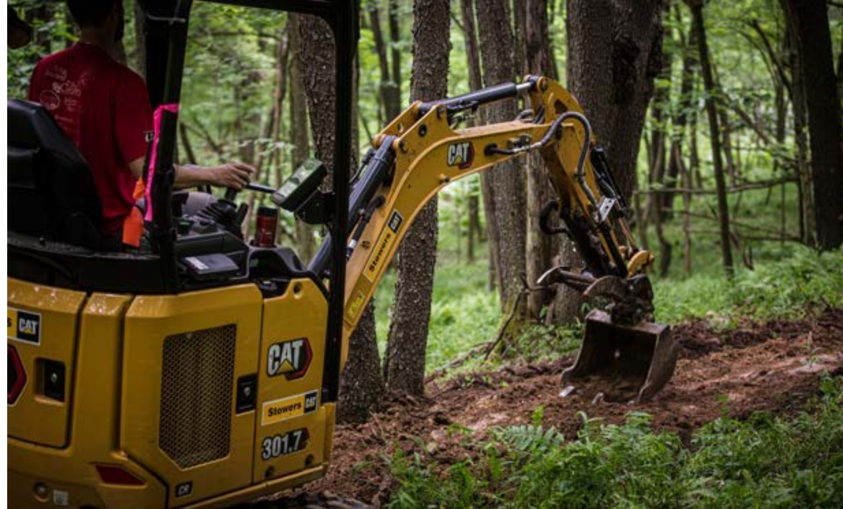
Mini excavator. Photo by Chrisman/IMBA
