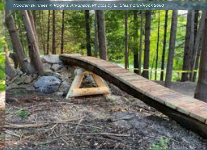
Chainsaw-milled wooden skinny alternate line at Blackhawk Ski Area in Madison, Wisconsin. Photo by Chad Landowski/Traction Trailworks
