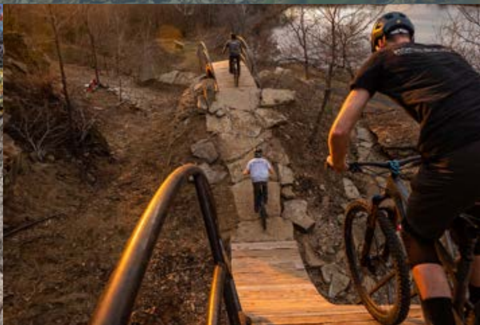
Custom designed and engineered roll-down trail feature in Vian, Oklahoma. Photo by Eli Glesmann/Rock Solid
