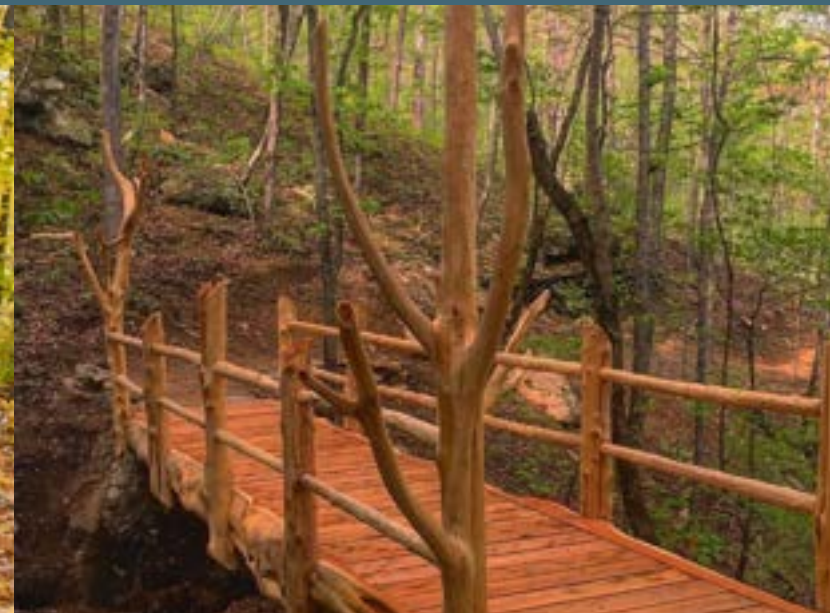
Hand-felled, hand-peeled, and hand-sanded bridges have a unique custom feel. Photo courtesy of Rock Solid
