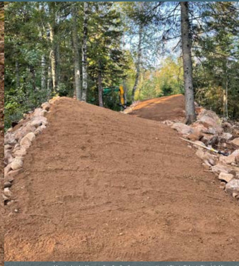
Monster banked berm rollers (rollers) pre-compaction at Giants Ridge in Biwabik, Minnesota. Photo by Adam Buck/Pathfinder Trail Building
