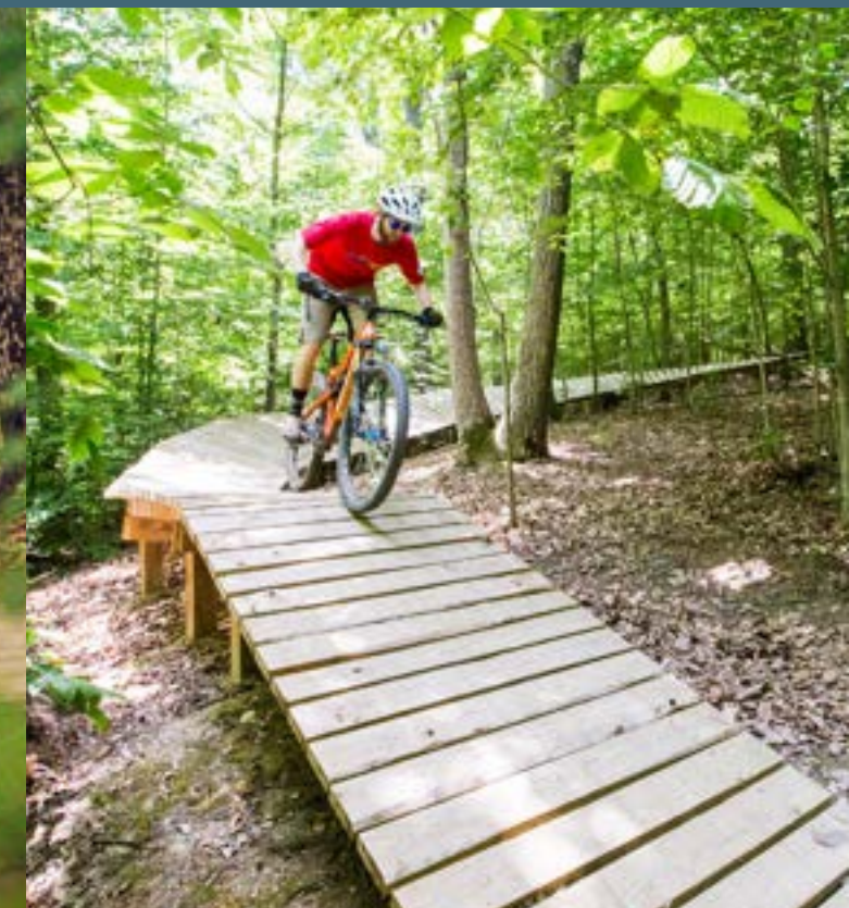
Wooden boardwalk with a canted turn for bike optimization. Photo courtesy of BLM/IMBA
