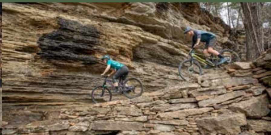
Intricate retaining wall at Devil's Den State Park in Winslow, Arkansas. Photo by Eli Giesmann/Rock Solid
