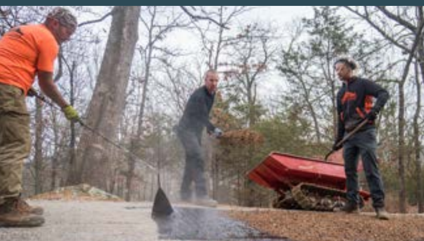
Liquid asphalt and final aggregate coat being applied at Centennial Park in Fayetteville, Arkansas. Photo by Eli Glesmann/Rock Solid
