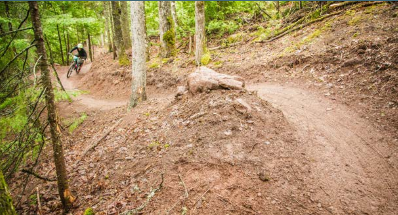
Insloped tread maximizes traction and flow. Photo by Hansi Johnson
