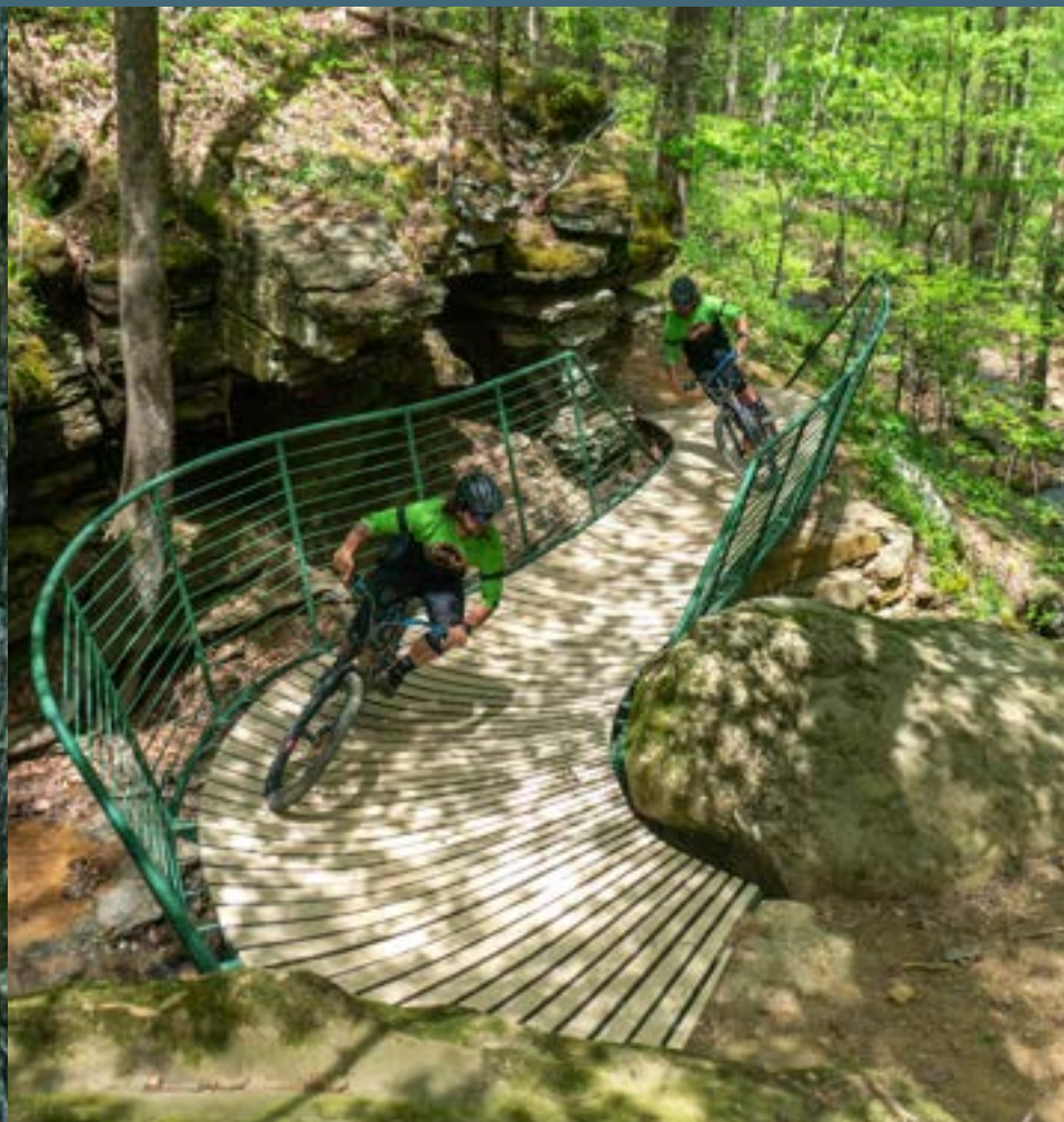
Complex, custom-engineered and site-built steel framed bridge at Mount Nebo State Park in Dardanelle, Arkansas. Photo by Andy and Michelle Flietstra/Rock Solid
