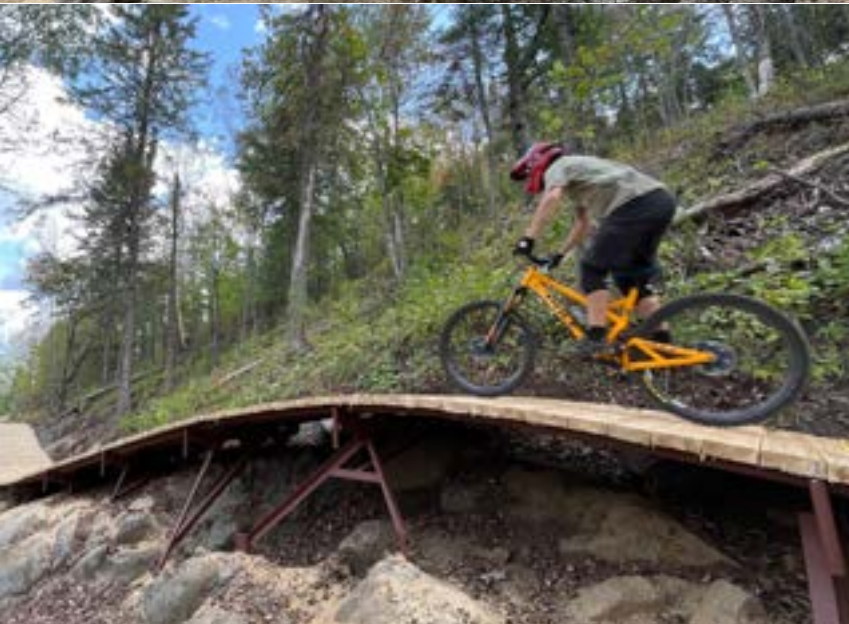
Custom steel-frame boardwalk with wooden decking at Giants Ridge in Biwabik, Minnesota. Photos by Adam Buck/Pathfinder Trail Building
