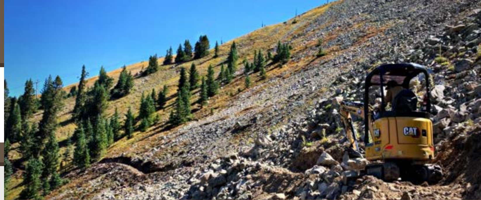
Excavator work at Arapahoe Basin, Colorado. Photo courtesy of IMBA
