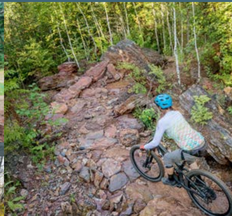
Constructed technical rock tread at Tioga Recreation Area in Cohasset, Minnesota. Photo by Chris Guibert/Rock Solid
