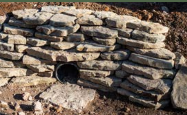
Small retaining wall with culvert. Photo by Eli Giesmann/Rock Solid
