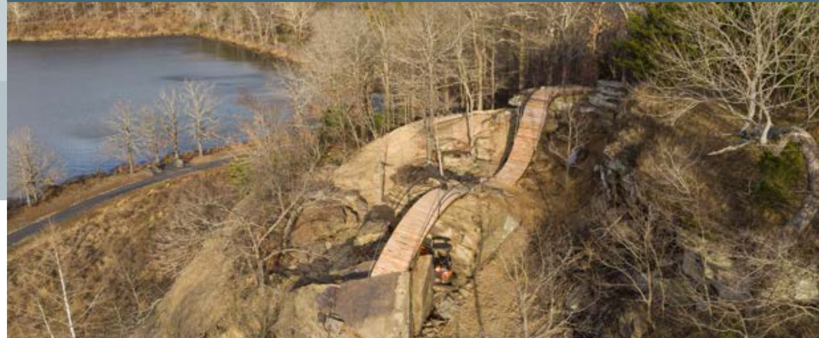
Custom designed and engineered trail feature at Lake Vian in Vian, Oklahoma. Photo by Eli Giesmann/Rock Solid
