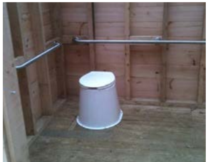
Accessible Toilet Riser and Stainless Grab bars. Also note clear T shaped turn around space.
