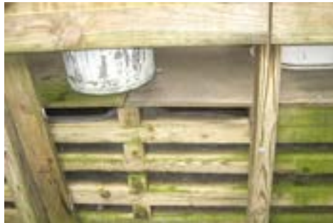
Moldering Crib - note plastic riser placement
