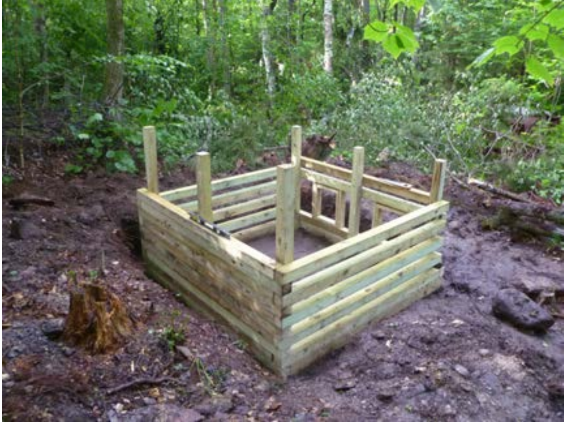
The completed moldering bin and six posts.
