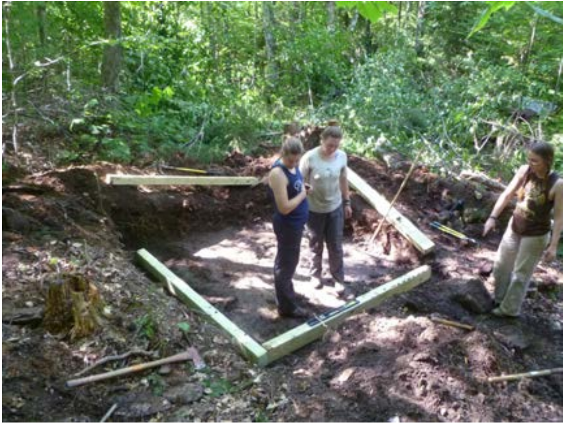
After digging out the site for the moldering bin.
