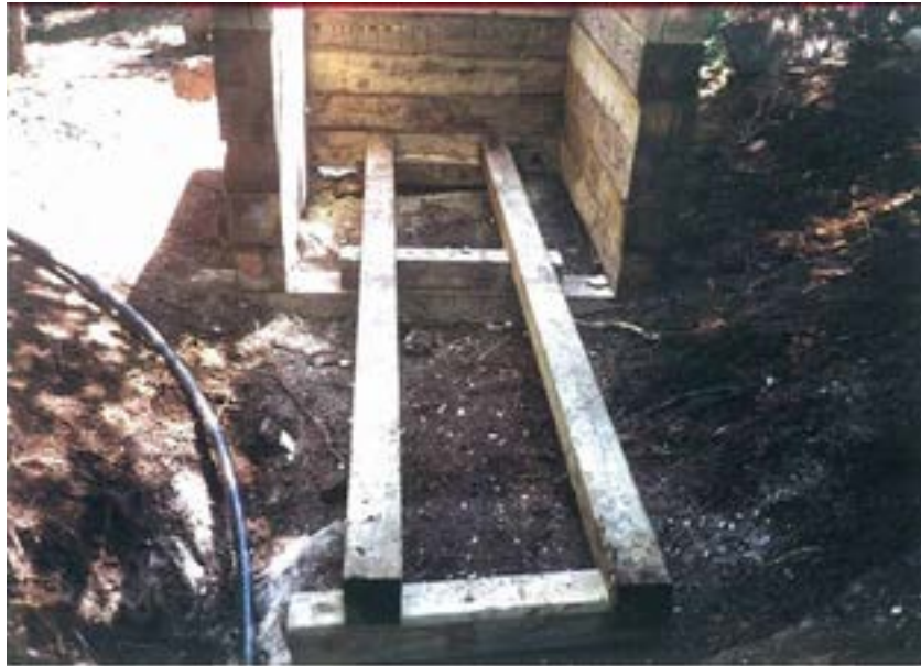
Rails for sliding out catcher - AMC
