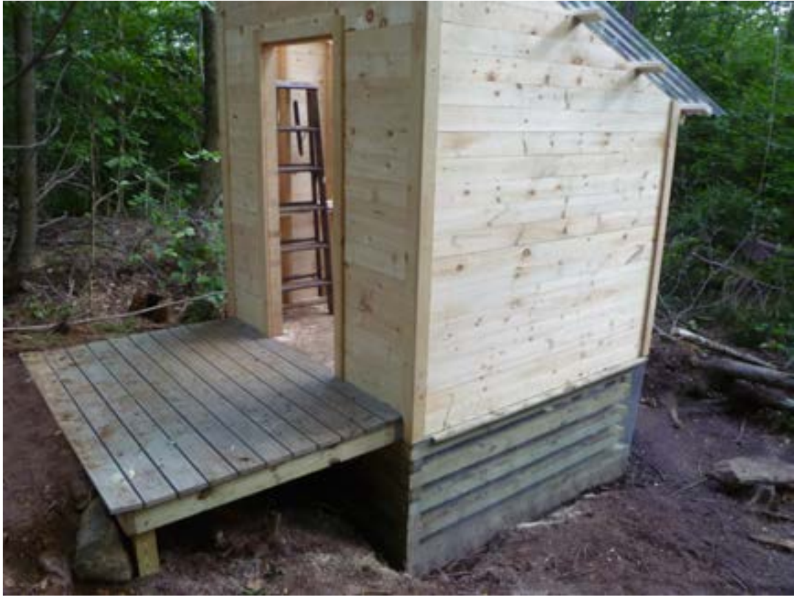
Siding and earth ramp added.
