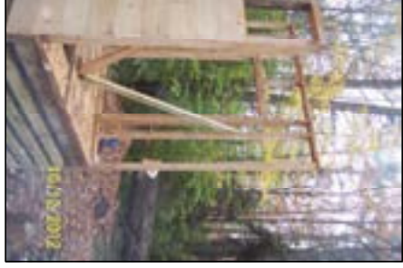
FRONT/BACK WALL BRACING
