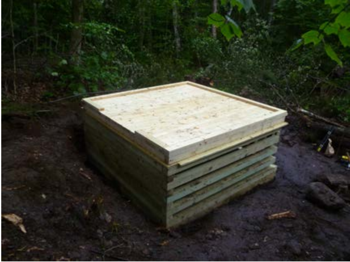
Completed floor and sill.
