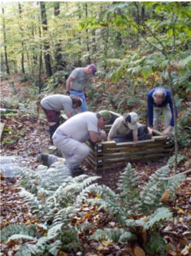
Photo #3. Lining the crib with screen.
