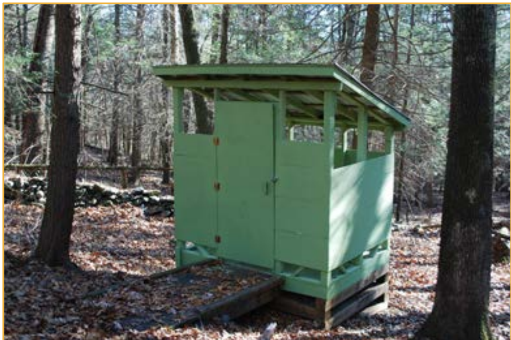
Moldering Privy with Accessible Ramp- A.T. Connecticut
