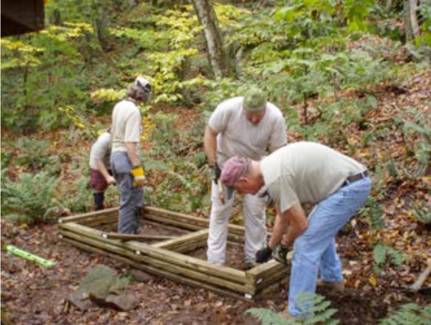
Photo #2. Crib assembly has begun.
