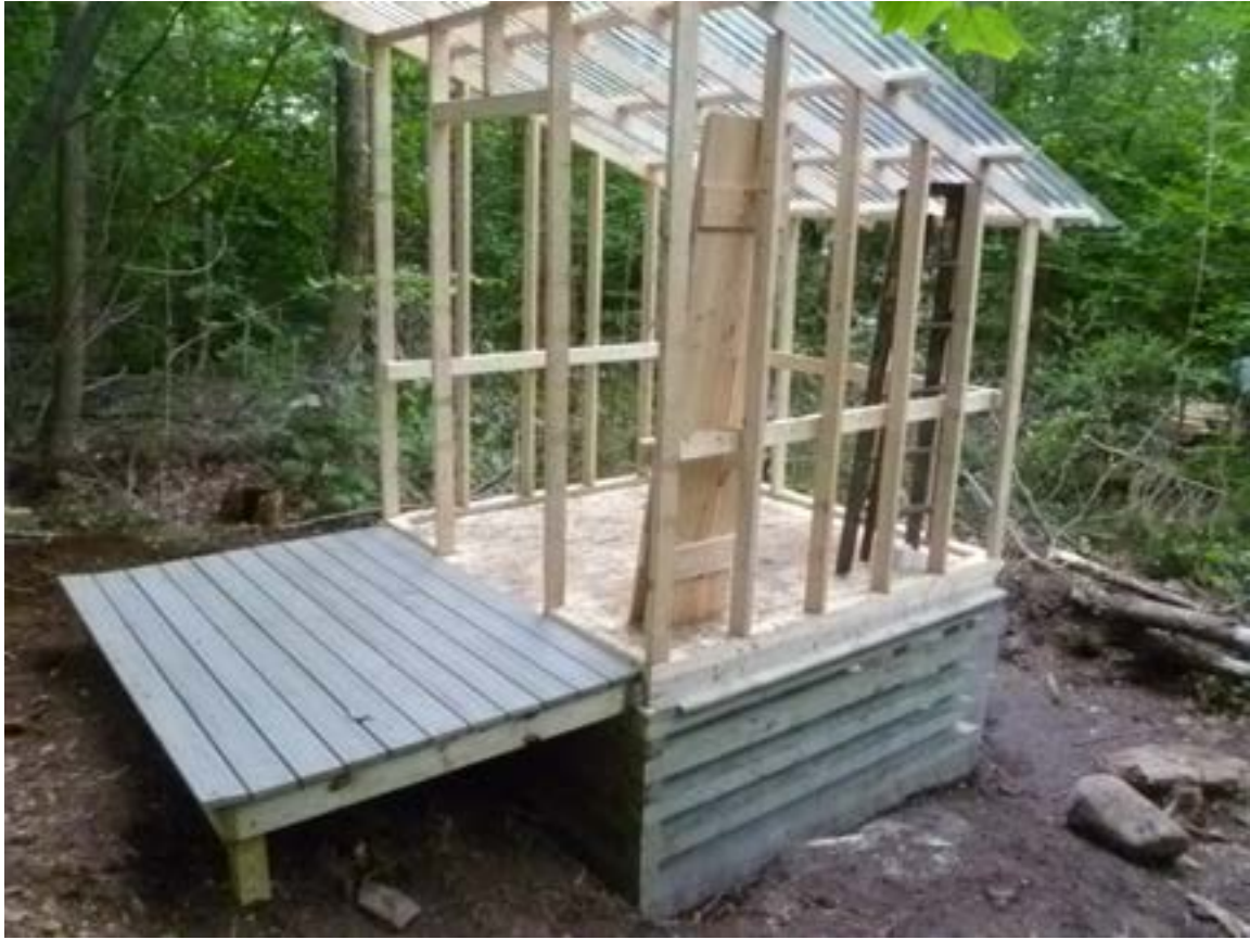
Roof and deck added.
