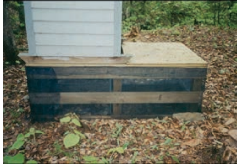
Double Chambered Moldering Privy Crib - note dark insect screening to help disguise the waste pile
