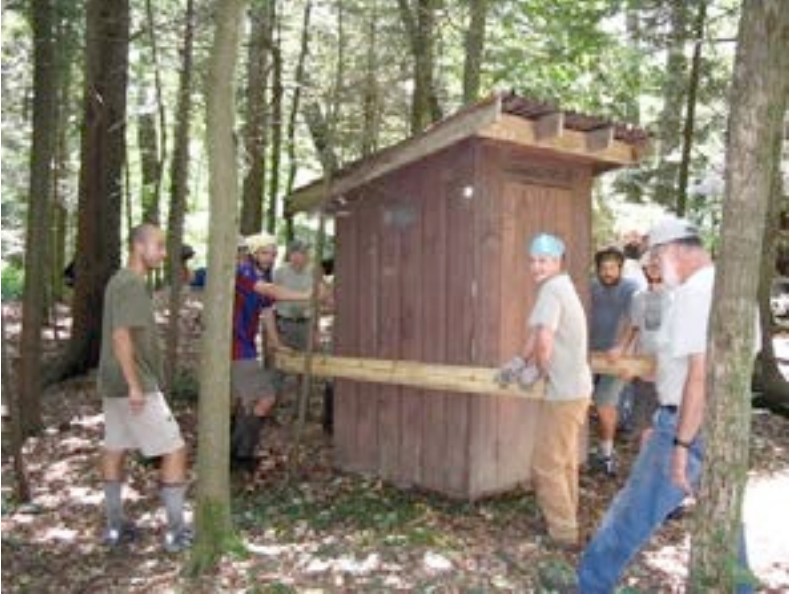
Photo #4. Existing outhouse ready to carry to crib location.
