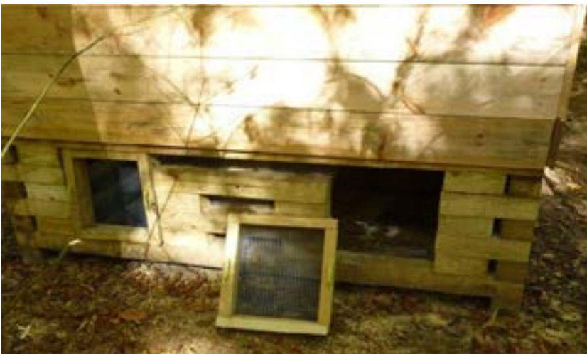
Access to waste pile is essential. Provisions must be made to do this without going through the toilet seat.
