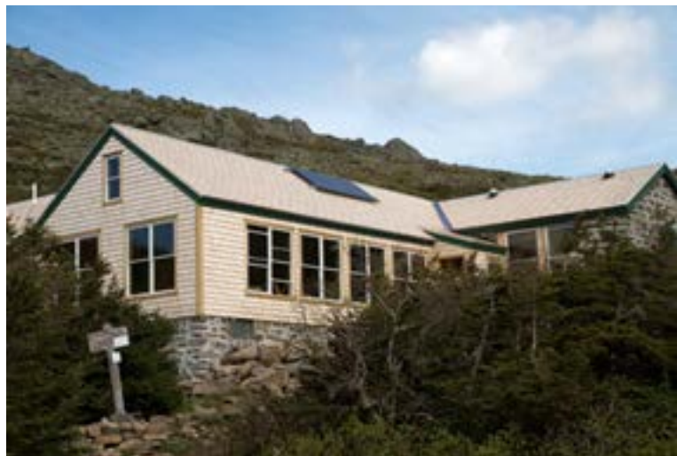
AMC's Madison Springs Hut utilizes a dewatering system
