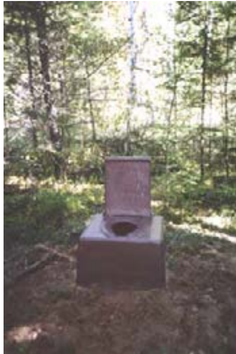
Figure 84—A fiberglass riser for a pit toilet in the Boundary Waters Canoe Area.
